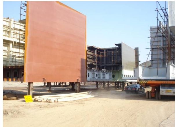
Section building and coating at Nantong Yahua Shipyard
