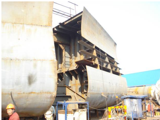
Bow section construction at Nantong Yahua Shipyard
