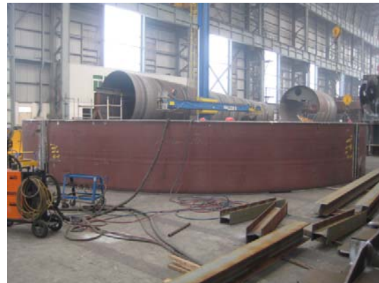
Huisman China, pedestal section foundation for lower slew bearing
