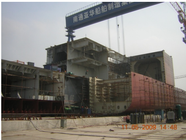
Hull section construction at Nantong Yahua Shipyard
