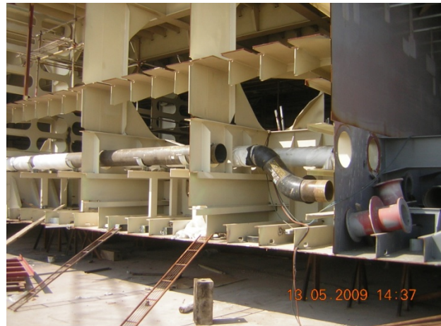
Piping assembly at Nantong Yahua Shipyard
